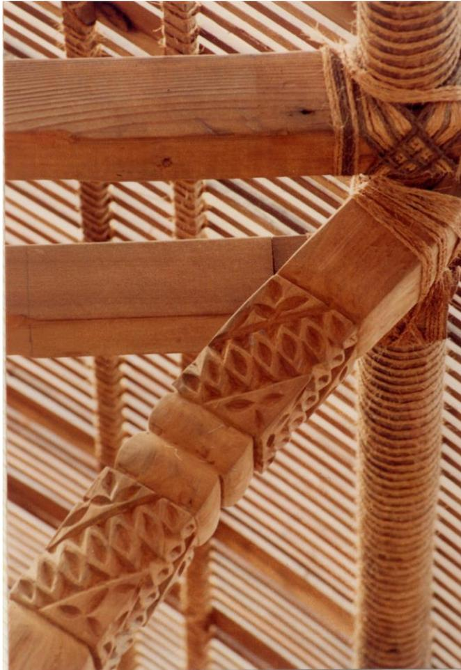
Traditional Samoan *fale* construction (roof beam detail)
